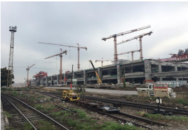
Red Line Construction Site
