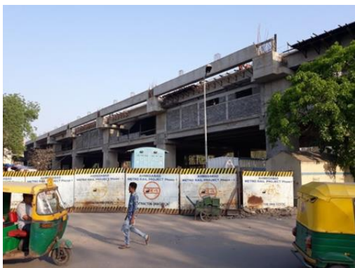
Station construction site where AFC will be installed
