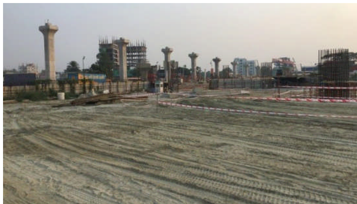
Construction Progress of Dhaka MRT Line 6
