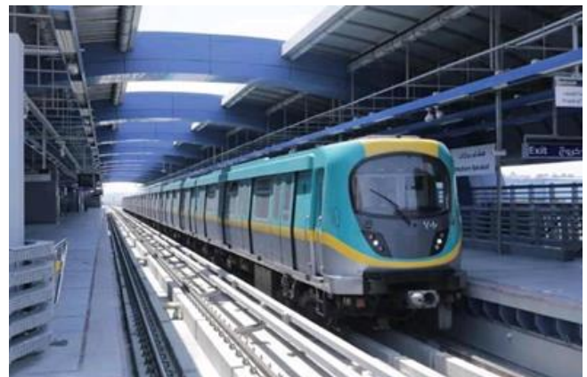
IMAGE : photo of Cairo Metro Line 3
