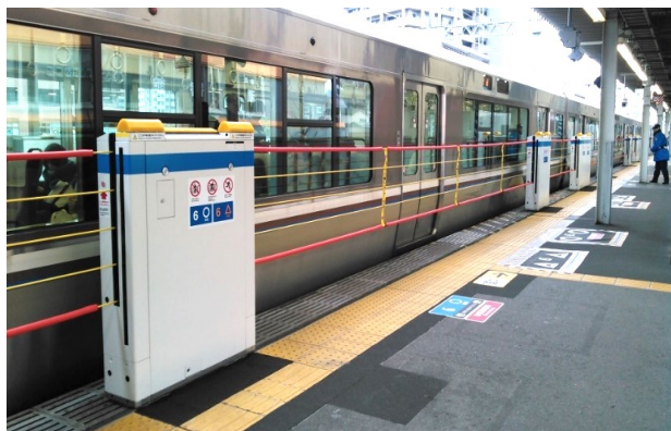
Wire-Rope Platform Screen Doors
